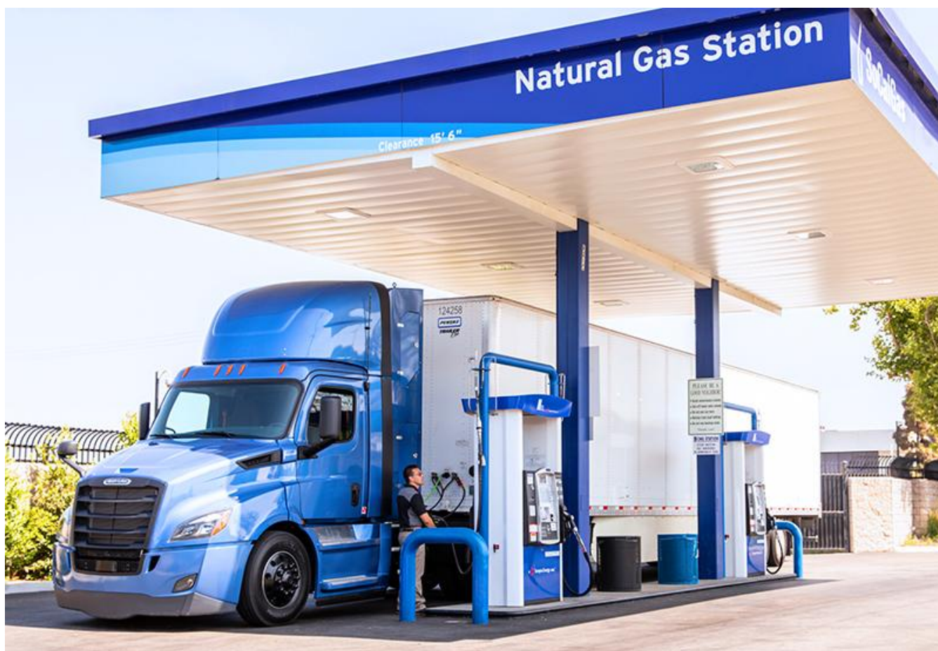
SoCalGas fueling station in California that dispenses RNG. Photo courtesy of SoCalGas
